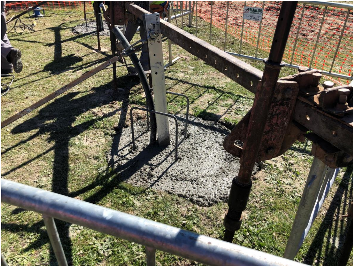
Concrete foundation of a pylon
